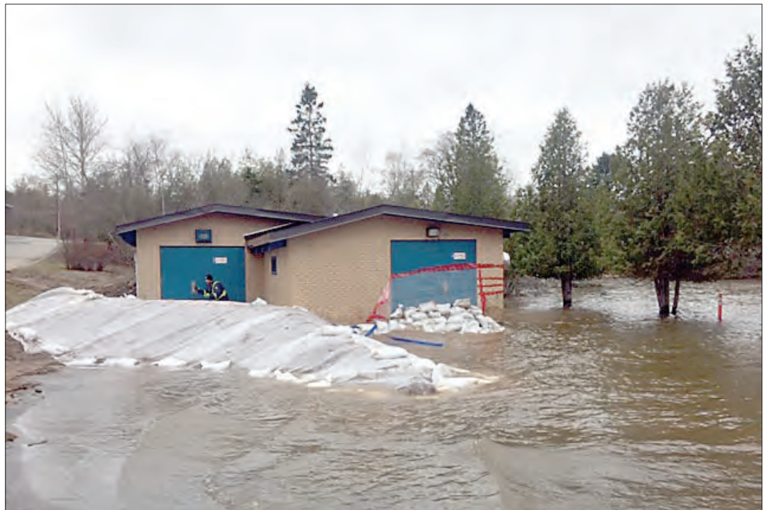
After viewing computer projections of just how much damage the flooding could do to Saint John's water and wastewater infrastructure in 2018, it was clear extra defences had to be put in place. The result was a construction of a clay berm around the wastewater plant in Millidgeville, which lay directly in the path of the rising waters.
