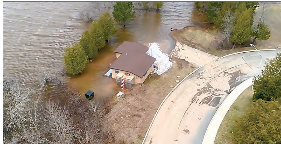
The berm was left in place and worked equally well this spring, when the water level again crested at just under six metres.
