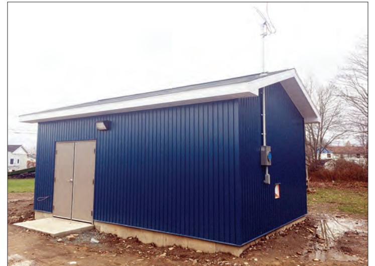
The new booster station built by the Town of Port Hawkesbury to service the Tamarac sub-division is one of two projects for the town to receive approval under the Clean Water and Wastewater Fund.
