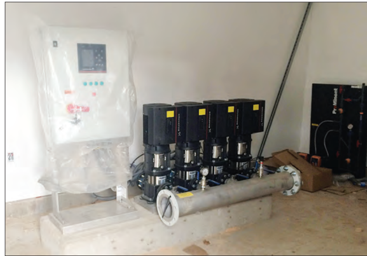
A new Grundfos pump package has been installed in the new booster station building that services the Tamarac sub-division in the Town of Port Hawkesbury. The project was one of two for the town to receive approval under the Clean Water and Wastewater Fund.
