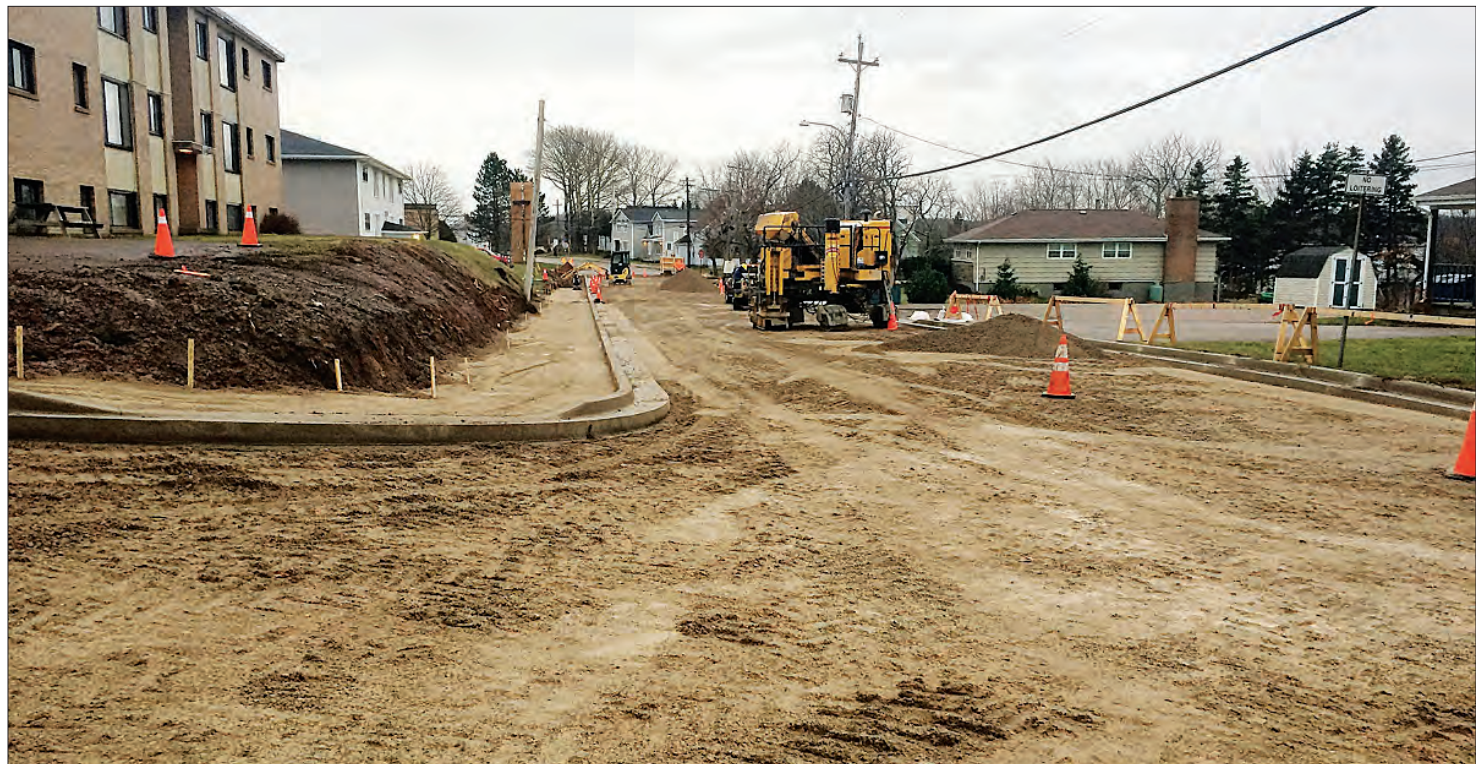
A $4.6 million street reconstruction project in the Town of Port Hawkesbury will see a total rebuild of both Pitt and Napean streets. Work was about 50 per cent completed before the winter weather set in. The project is expected to be completed this summer.
