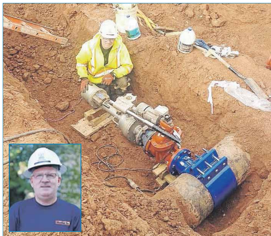
Blaine Parkman, water and sewer utility foreman with the City of Charlottetown, at work creating an eight-inch water main tap.
