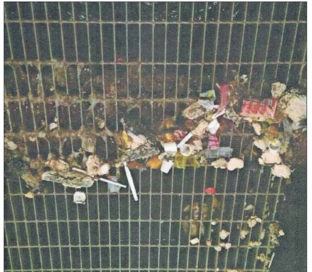
This is the material that the Public Works Department found on the rack when the jail's macerator was off line.
