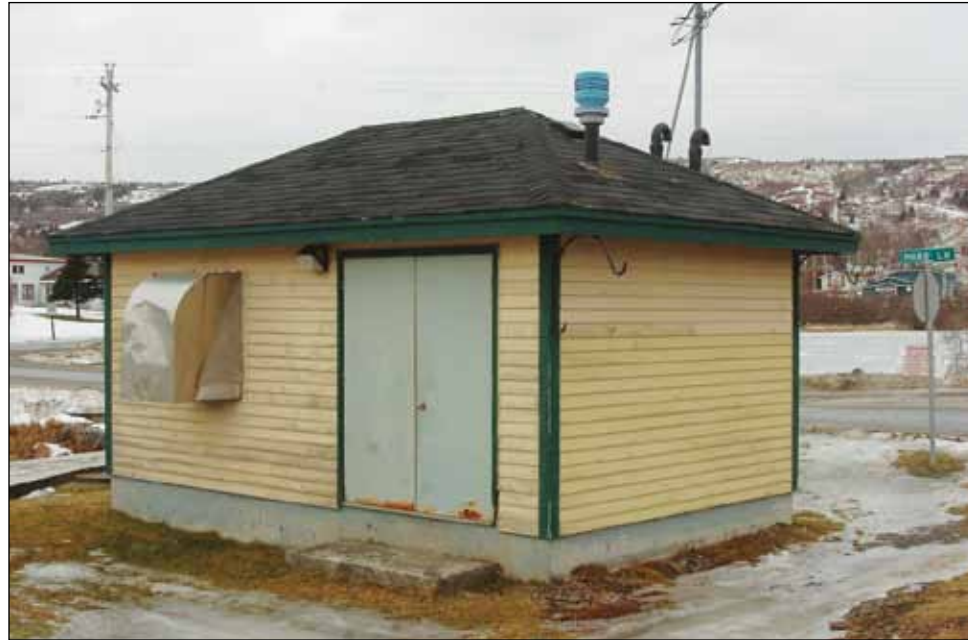
Planned upgrades for the lift station at the bottom of Pike's Lane in Carbonear, Newfoundland & Labrador will be going ahead, pending approval from the Department of Municipal Affairs on a tender that's come in well over the budgeted cost. (Photo: © Andrew Robinson/The Compass)
