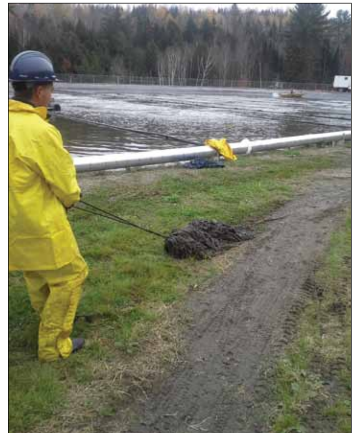
Wipes are removed from a treatment facility in Fredericton, New Brunswick in October 2014. (Photo: Courtesy of Neil Thomas)
