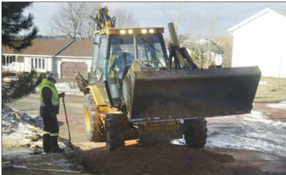
City workers make repairs to a Charlottetown water and sewer line Feb. 19 near Queen Street. The Prince Edward Island city's infrastructure is comprised of piping that varies in age from the newly installed in 2014 to the very old from 1888. (Photo: © Heather Taweel/The Guardian)
