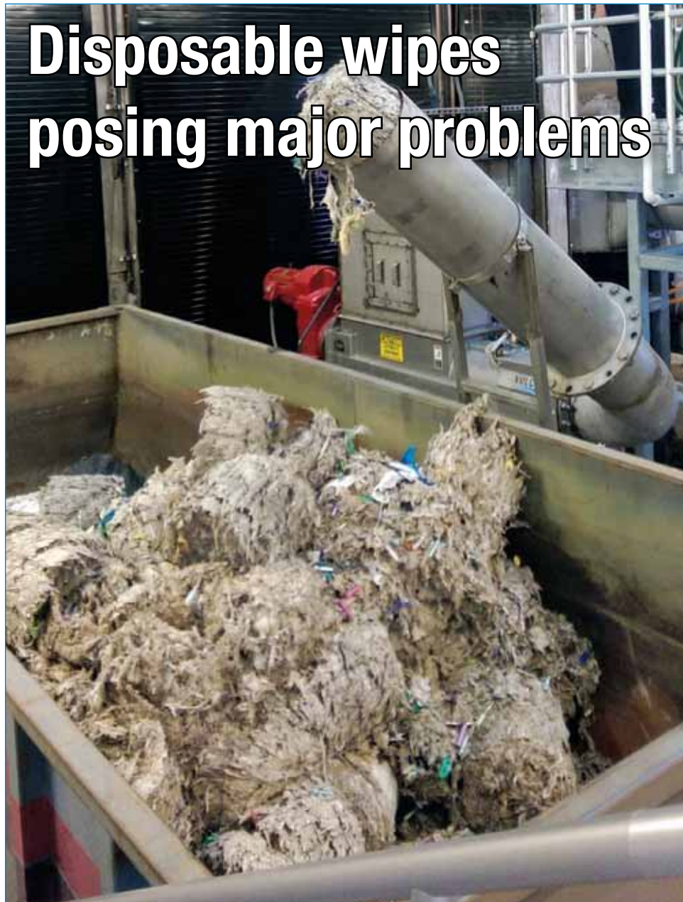
Disposable wipes and other debris fill a bin at this treatment plant. (Photo: Courtesy of Barry Orr)
