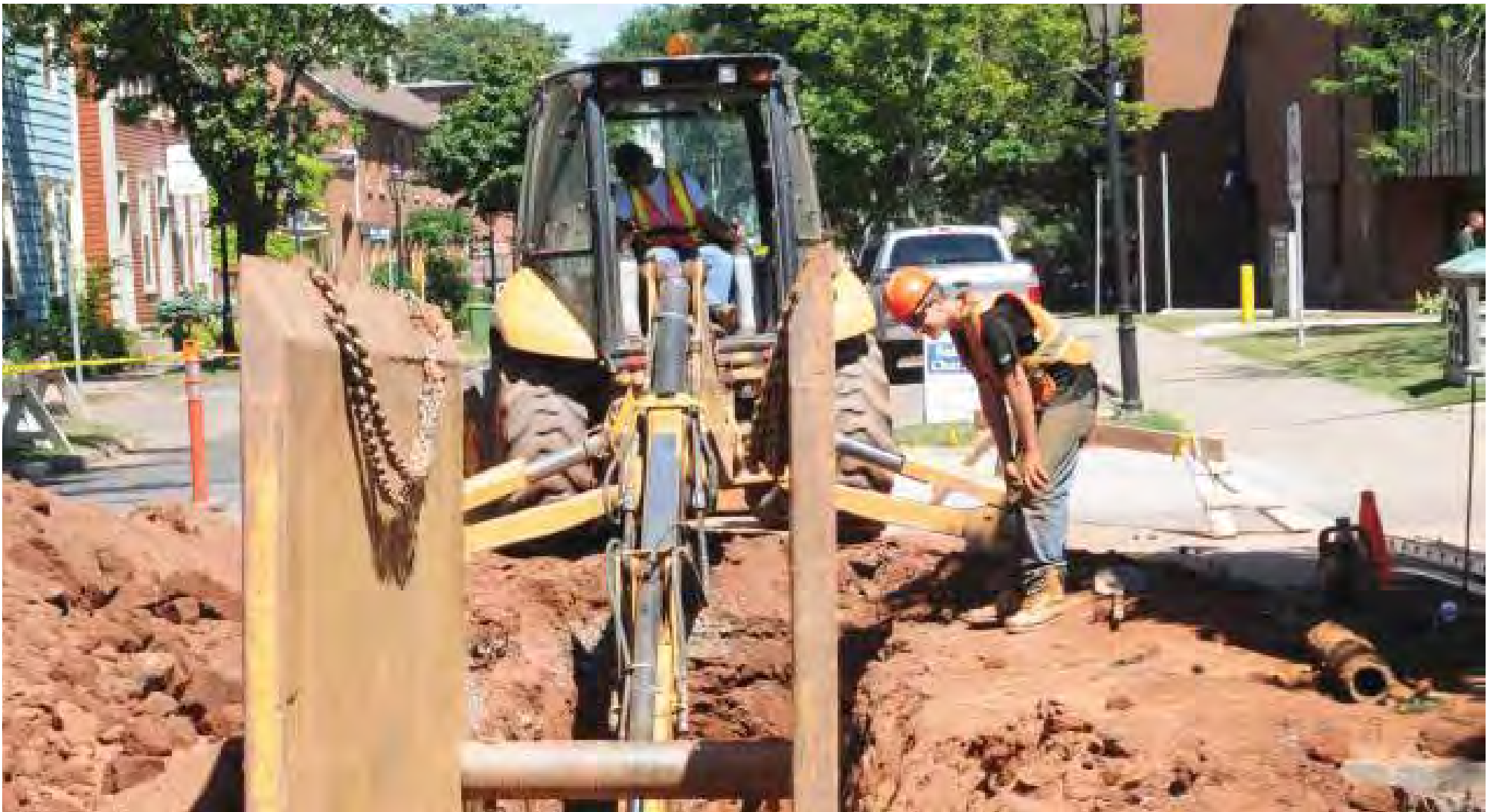
Construction is now underway on a major upgrade to Charlottetown's sewer system. (Photo: © The Guardian)
