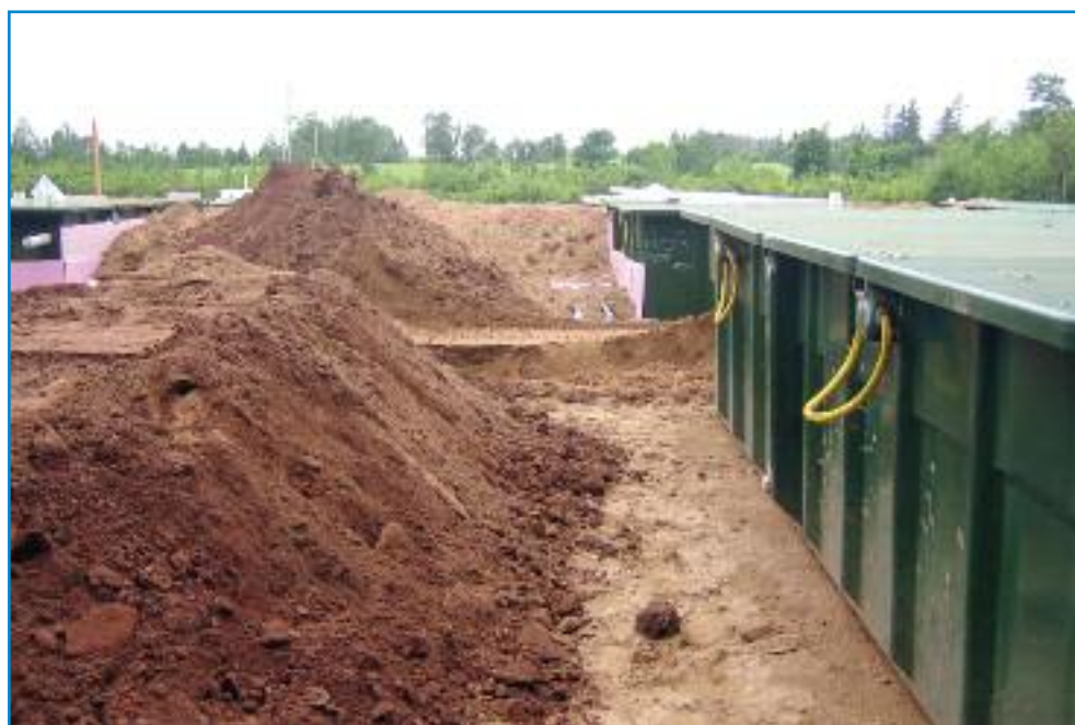
Ten modular AdvanTex AX-100 Textile Filters are installed in-ground and treat Victoria, Prince Edward Island's wastewater to better than secondary standards: below 10/10 BOD and TSS. (Photo: Courtesy of Orenco Systems®, Inc.)
