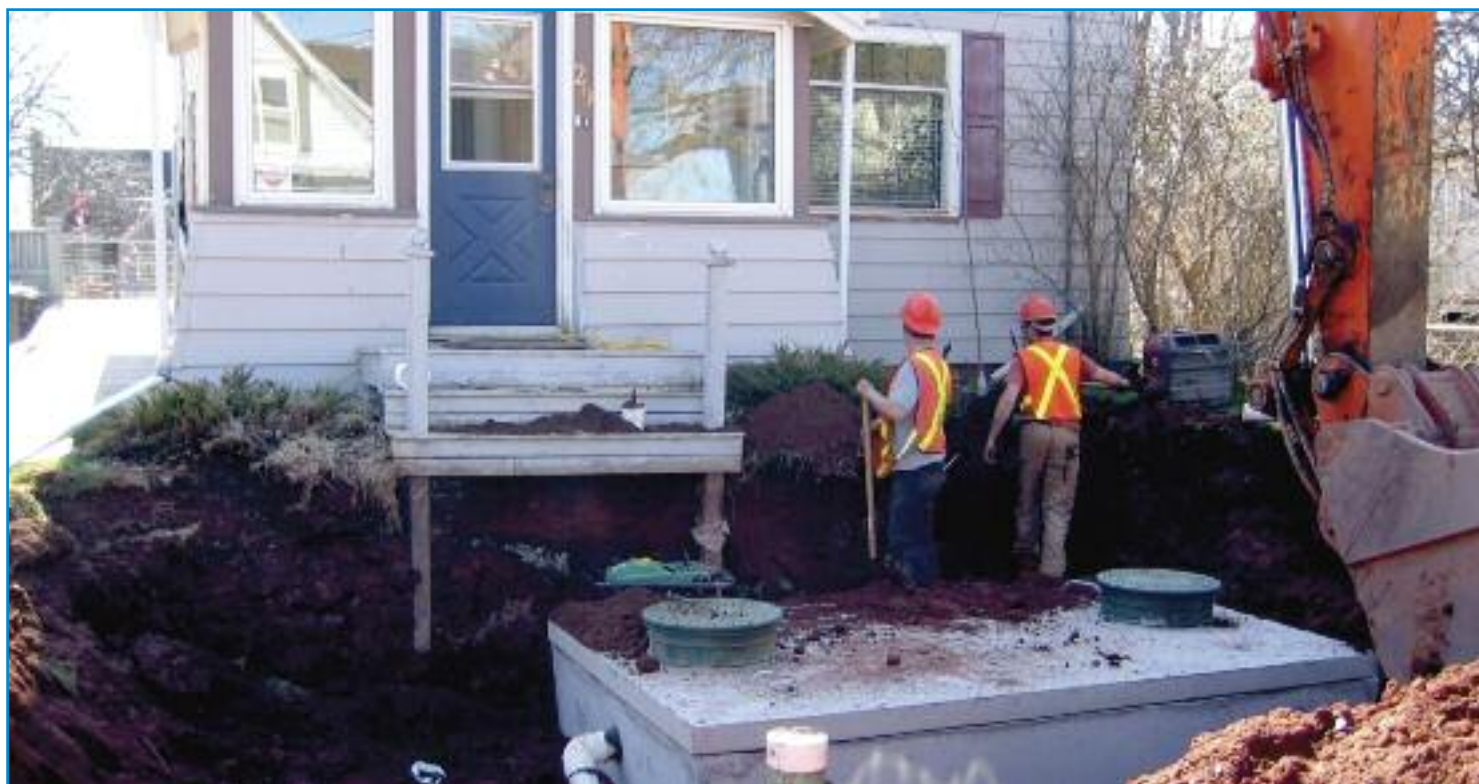
This photo shows the installation of a new onsite (on-lot) tank on one of the properties connected to Victoria, Prince Edward Island's new effluent sewer system. (Photo: Courtesy of Orenco Systems®, Inc.)
