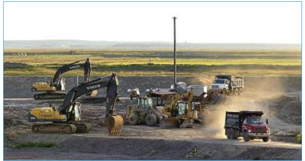
Amherst's $12-million sewage treatment plant is about a month behind schedule due to weather and other factors. (Photo: Dave Mathieson/ Amherst Daily News)
