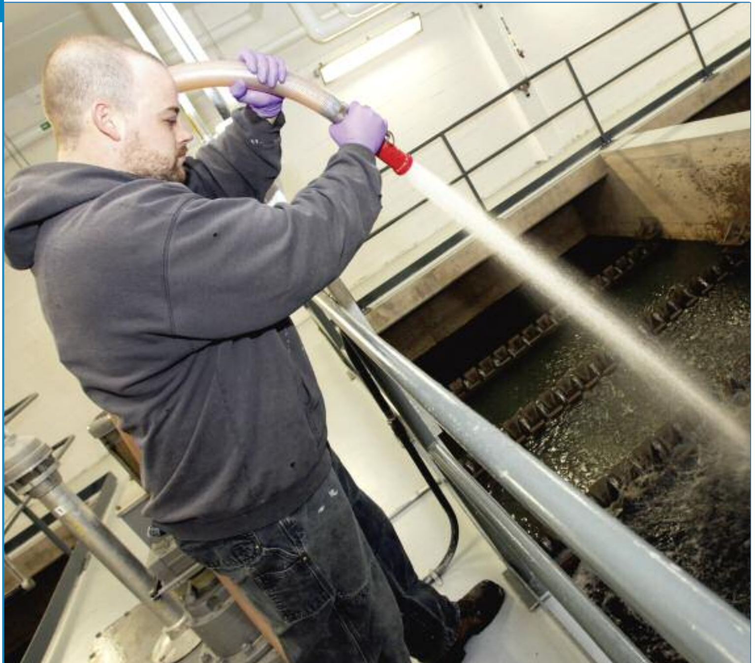
Jody Hawkins, a plant operator at the Battery Point municipal wastewater treatment facility in Sydney, Cape Breton, Nova Scotia sprays clean water into a clarifying tank — agitating the human waste and cleaning excess debris from the system to keep it flowing freely. The clarifying tanks are part of the treatment process that separates solids from water in the waste material. (See story on page 8) (Photo: Steve Wadden/Cape Breton Post)
