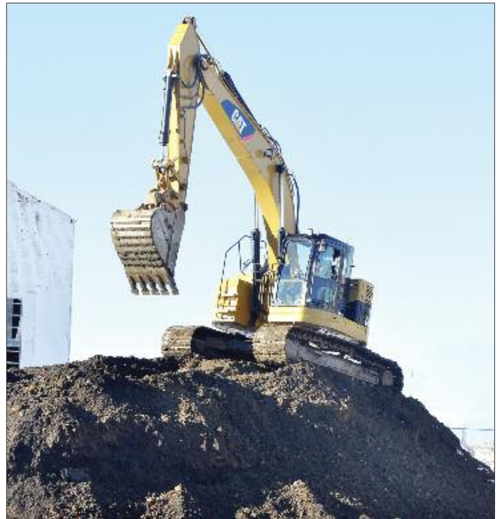
This lot along Main Street in Trenton, Nova Scotia was a hive of activity on Jan 17 as work began on Phase 2 of the pumping station upgrade project. (Photo: Ray Burns/The News)
