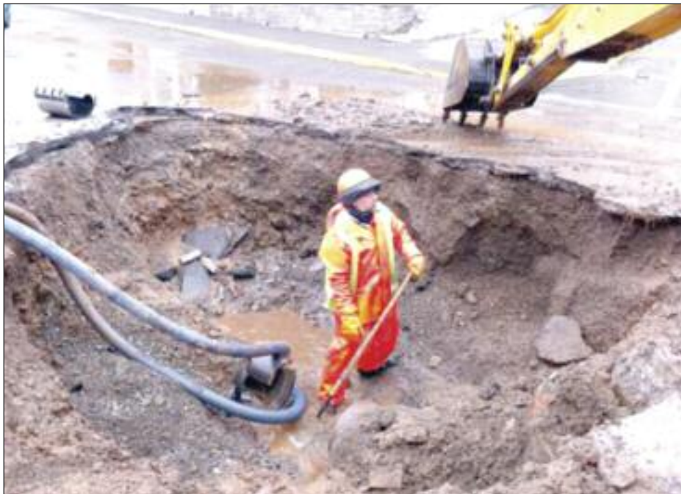
Public work crews were on the scene early on Church Street in New Glasgow, Nova Scotia on March 8 trying to repair a water main break. One town worker said he noticed the break at about 2 a.m. on his way to work. He said both the backhoe and a town truck sunk into the ground where the break occurred. The truck had to be pulled out of the hole. (Photo: Sueann Musick/The News)
