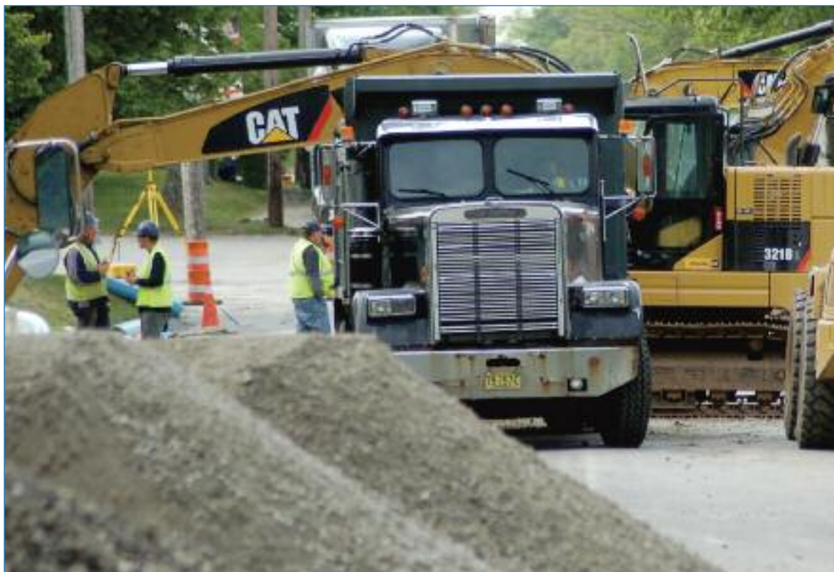
Construction is underway in Shelburne, Nova Scotia on the $2-million (plus) extension of the town's waterline. (Photo: Greg Bennett/The Coast Guard)
