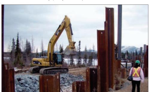
This picture taken at the Mushuau Innu First Nation community of Natuashish, Labrador shows Phase I (left) and Phase II (right) of the four-phase steel pile shoring excavation to extend twin water intake pipes from the existing pumphouse to Sango Brook seen in the background. (Photo courtesy of Indian and Northern Affairs Canada)
